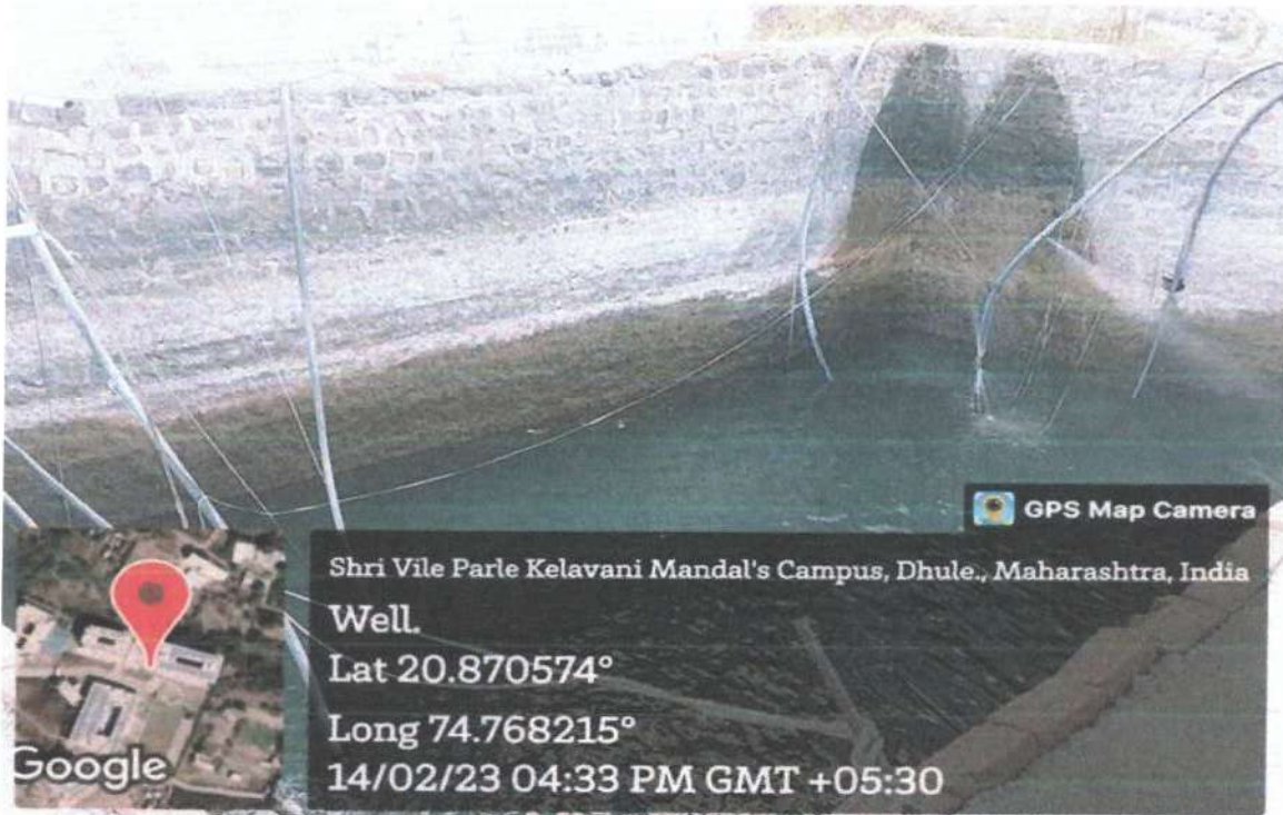
Photo of Open well recharge
