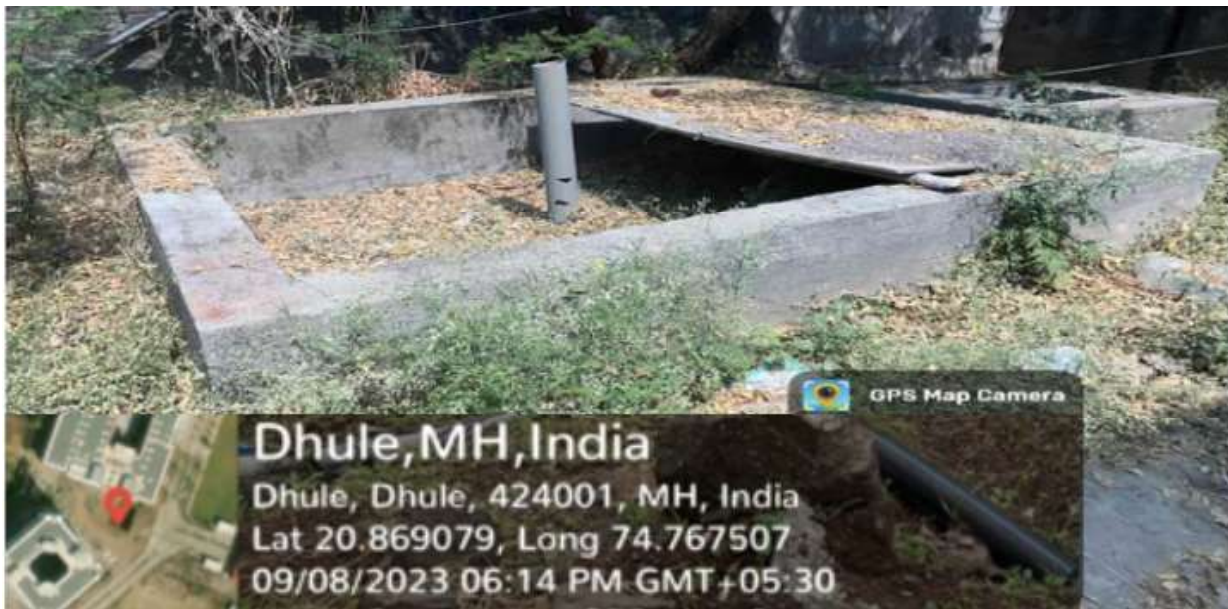
Rainwater harvesting recharge pit
